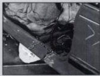
The two halves were then welded together at the windshield posts, at the rocker panels and under the carpeting. Now only minor repainting is needed to hide the fact that this is two cars spliced together.
